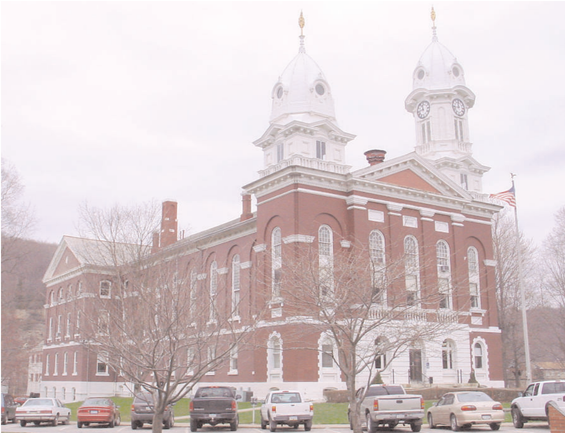
Figure 5: Venango County Courthouse
