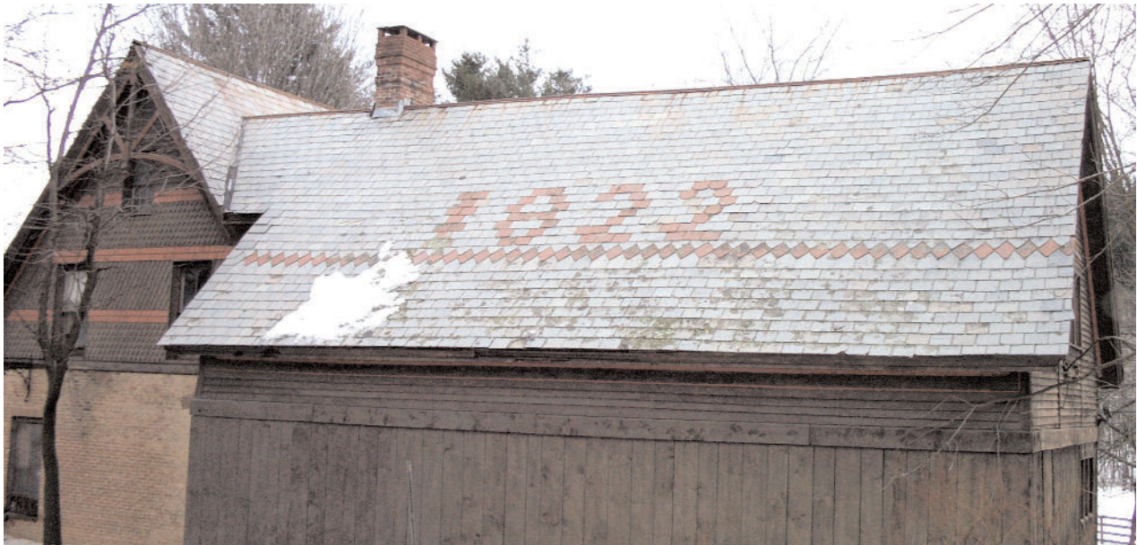
Figure 1: A recent photo of a barn in Vermont testifies to the potential longevity of a standard slate roof.
