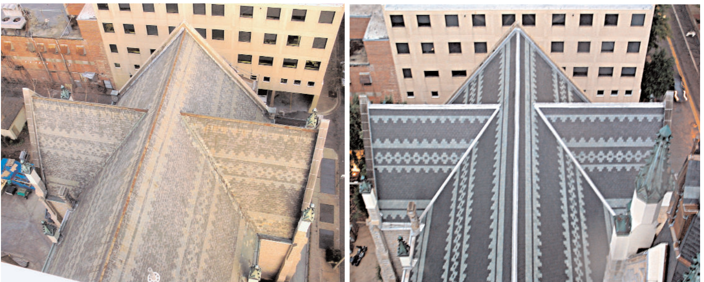
Figure 7: The Cathedral of St. Andrew in Little Rock, Arkansas, had worn out its black Pennsylvania slate after 120 years (above left). The Cathedral's new roof, installed by Midland Engineering in 2003, is likely to last 150 years. Vermont unfading green slate mixed with Welsh black slate and terne-coated stainless steel flashings should out-perform the original roof. Left photo by Joseph Jenkins; right photo by Lyle Bandurski.
